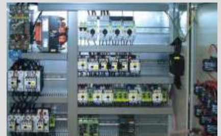
Integrated control panel for easy set-up (Plug & Play)
